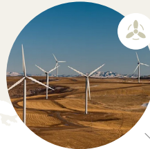
Gansu Guazhou Beidaqiao No.4 Wind Farm Project 中国本土 2,189 MWh
